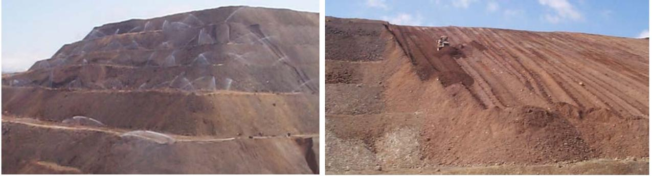
**Figures 2 and 3: Side slope leaching then re-sloping a Carlin-type ore heap.**
