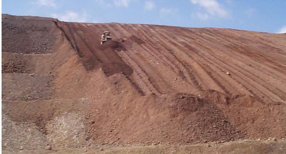
**Figure 5: The dozer side-slope contouring of a Carlin-type heap-leach operation (Seal, 2003).**
